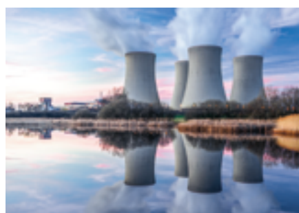
Specialised Fabrication Assemblies in Nuclear
