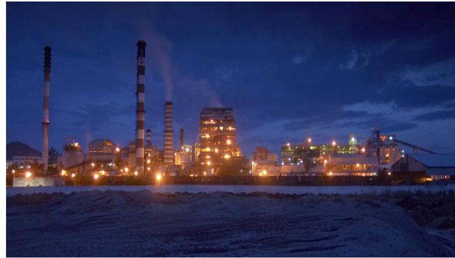
Panoramic view of the Unit JKPM (in Odisha)
