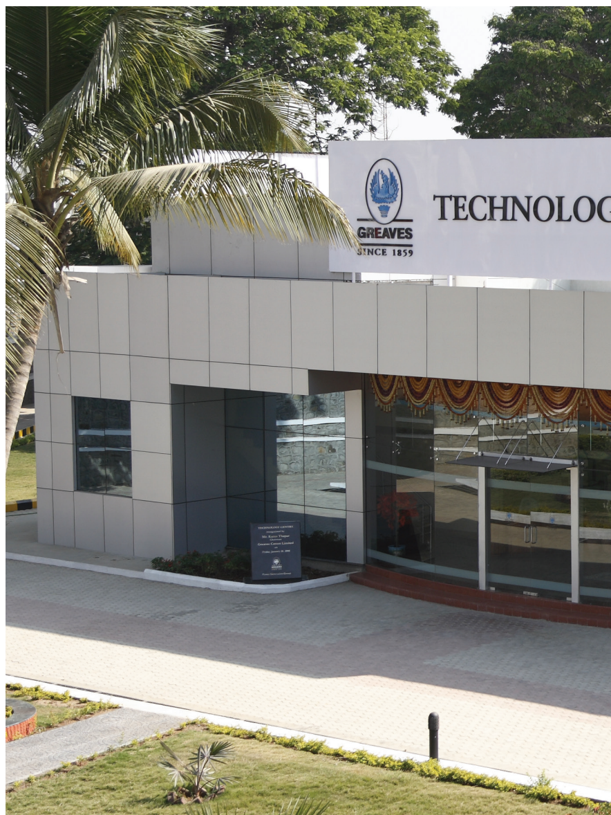
Greaves Technology Centre, Pune, Maharashtra
