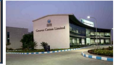
Technology Centre at Aurangabad
