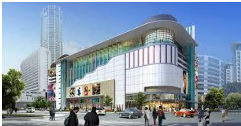
Retail, Hotels, Hospital & Commercial Complexes
