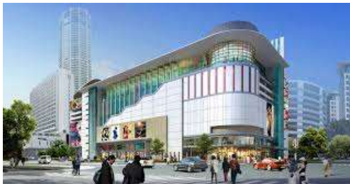
Retail, Hotels, Hospital & Commercial Complexes
