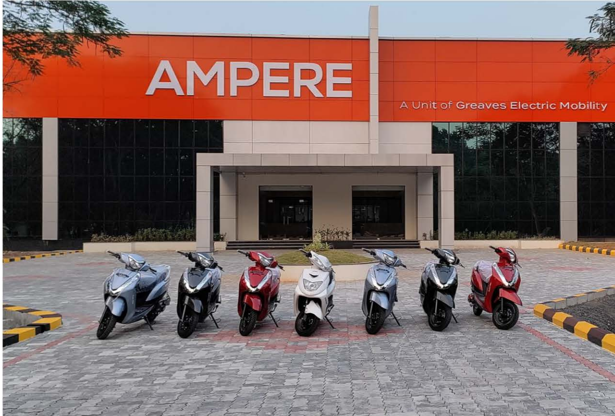
Ampere Manufacturing Facility, Ranipet
