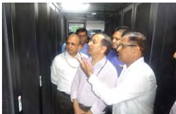
ML-Railway Board visit at Gurgaon Data Center
