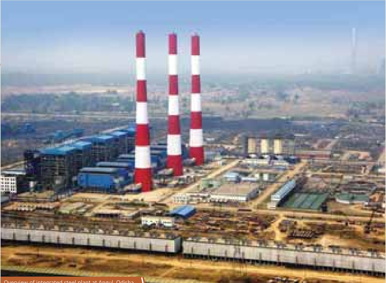
Overview of integrated steel plant at Angul, Odisha
