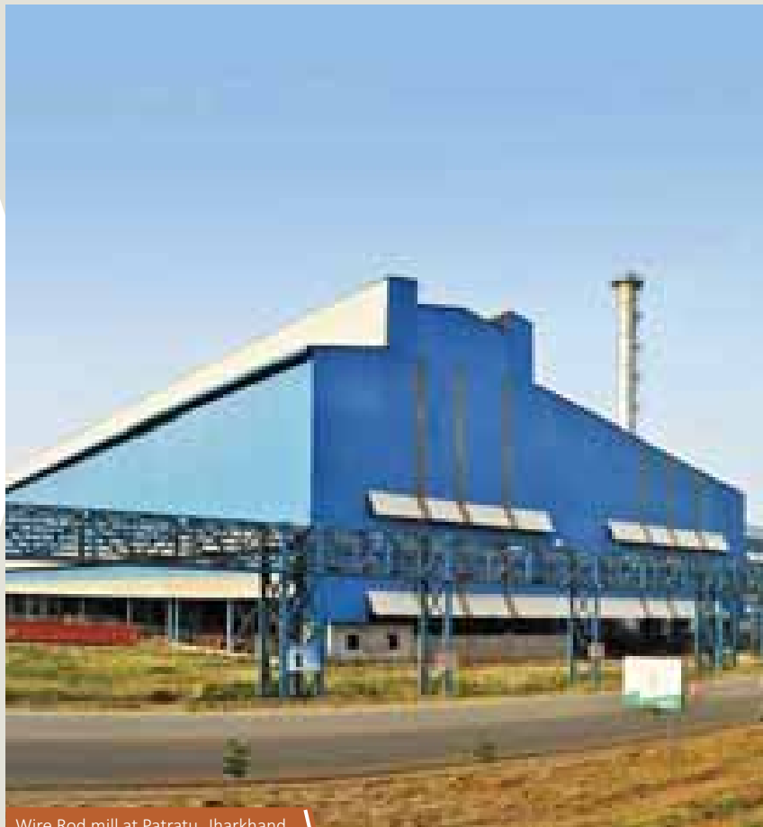
Wire Rod mill at Patratu, Jharkhand
