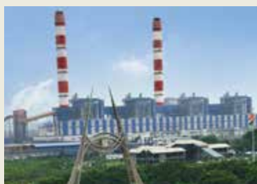
India's First Mega Power Project of 1000 MW in private sector at Tamnar, Chhattisgarh
