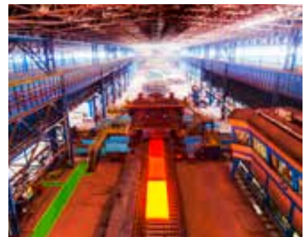
▶ 1.2 MTPA Plate Mill at Angul, Odisha
