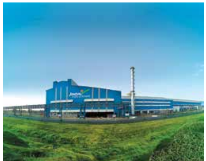
> 1 MTPA Rebar Mill at Patratu, Jharkhand
