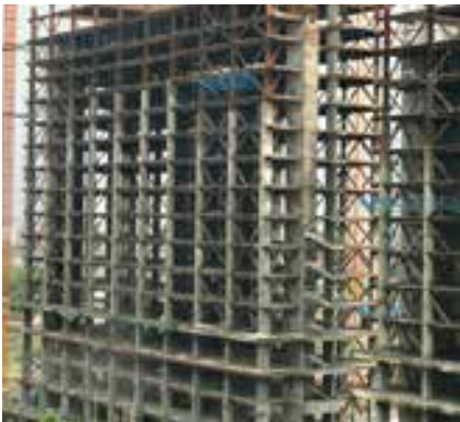
▶ High Rise Steel Buildings
