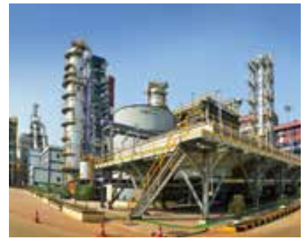
World's biggest Syn Gas based DRI plant at Angul, Odisha
