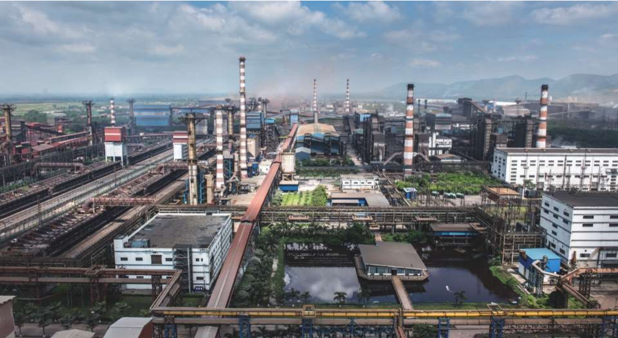
Aerial View of Raigarh Plant
