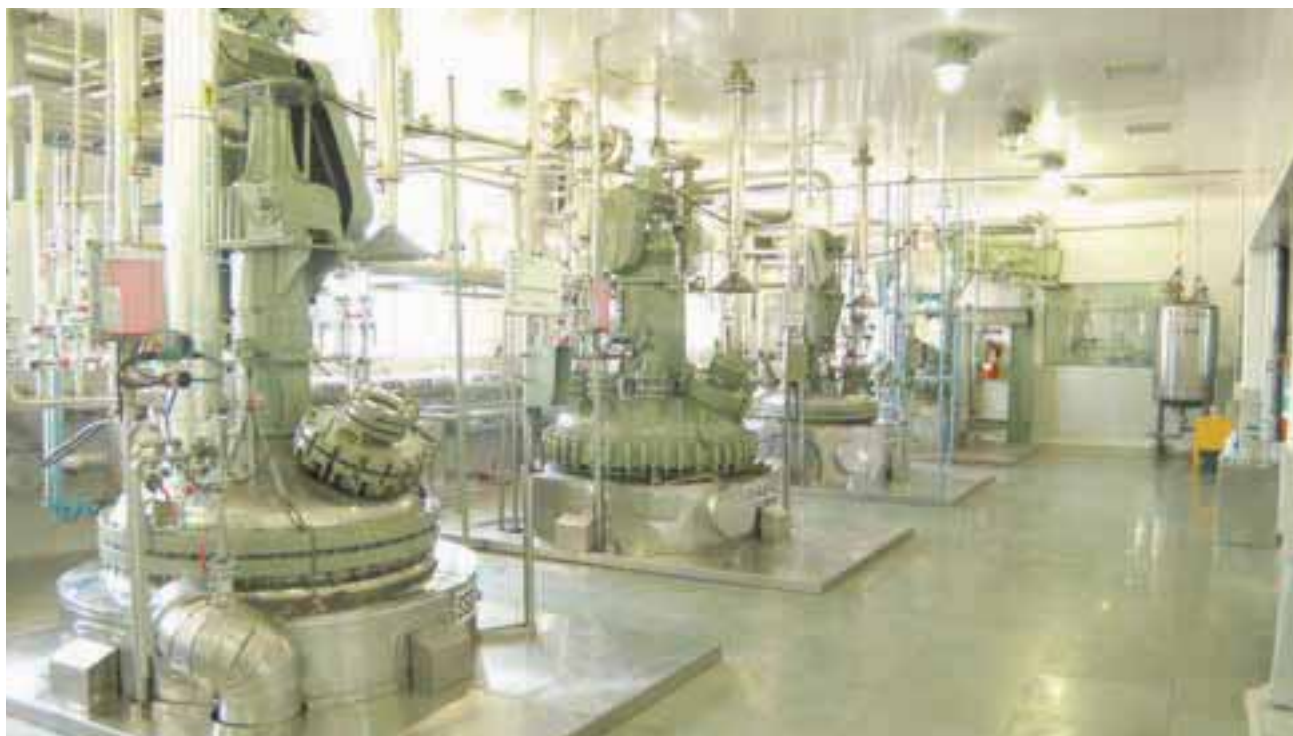
A snapshot of Glenmark's API Manufacturing facility in Ankleshwar, India
