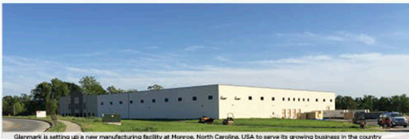
Glenmark is setting up a new manufacturing facility at Monroe, North Carolina, USA to serve its growing business in the country
