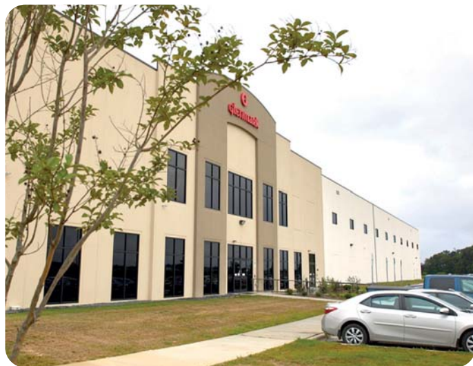
Glenmark's manufacturing facility at Monroe, North Carolina, US
