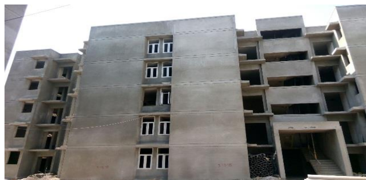
Happinest Boisar – Building B3 (Dec'15)
