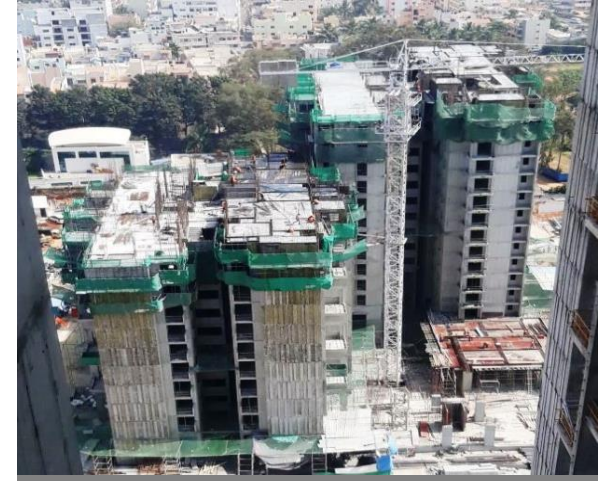
Windchimes II -Tower III&IV (Dec'17)
