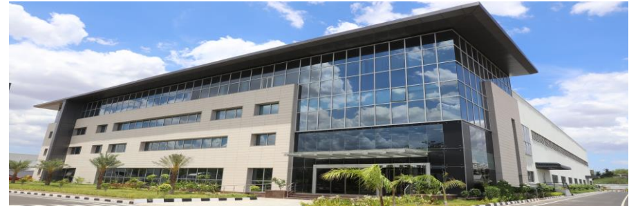
Dorma Kaba facility in DTA
