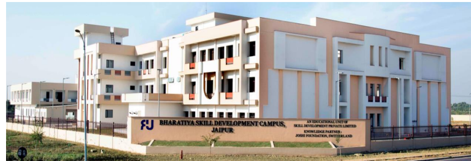
Bharat Skill Development University facility in DTA
