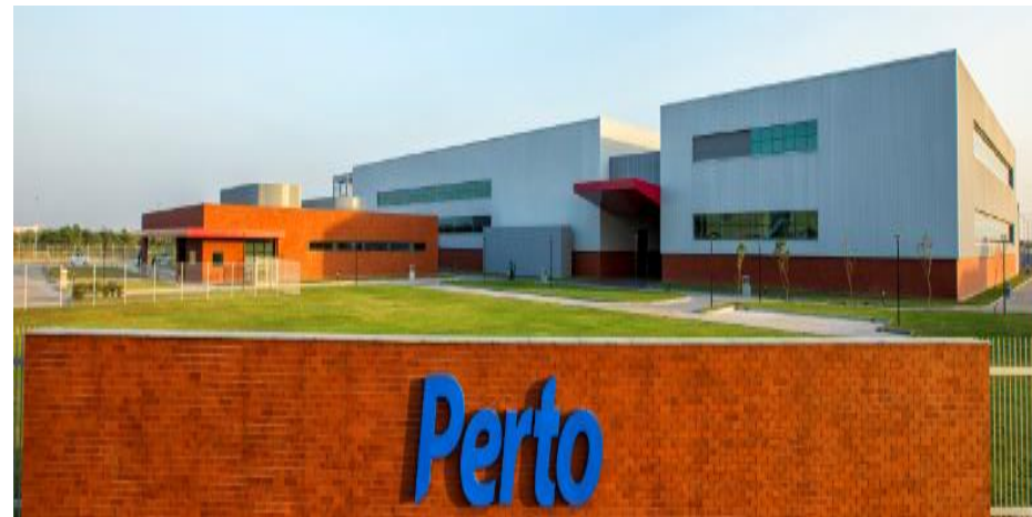
Perto facility in DTA
