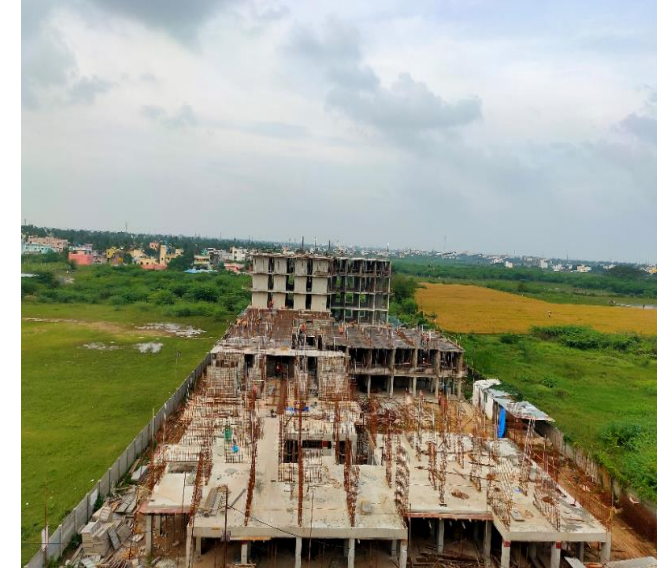
Happinest Avadi: Site under construction
