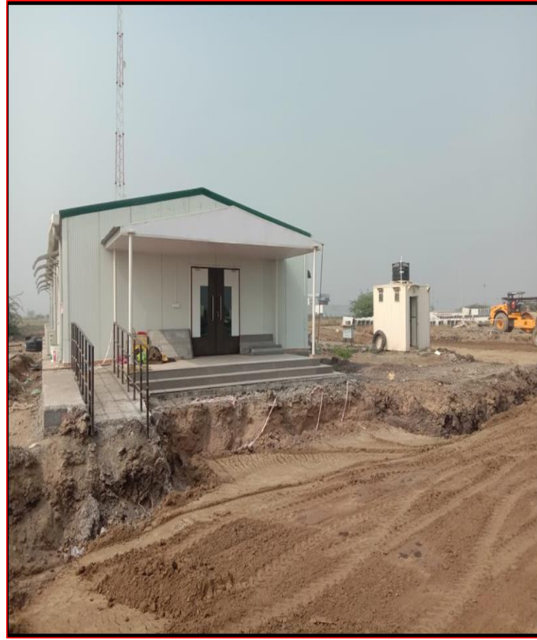
Site Under construction, Ahmedabad
