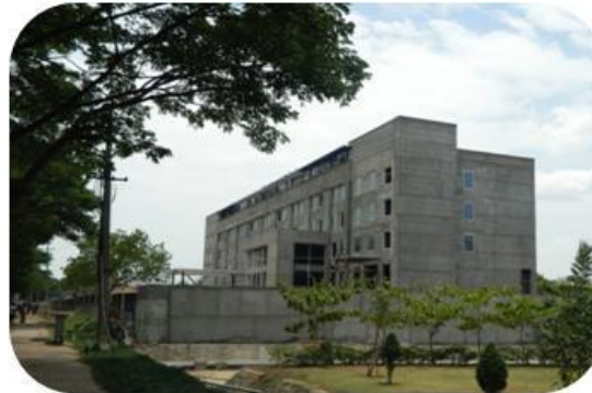
HolidayInn Express ( Under construction )
