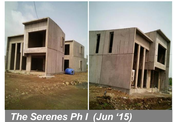
**Note:** Units constructed using precast technology
