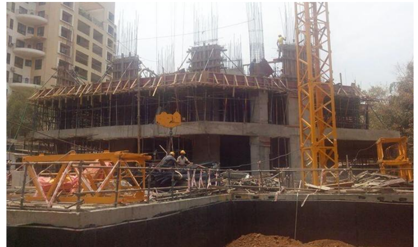
Construction Progress (Mar'14)
