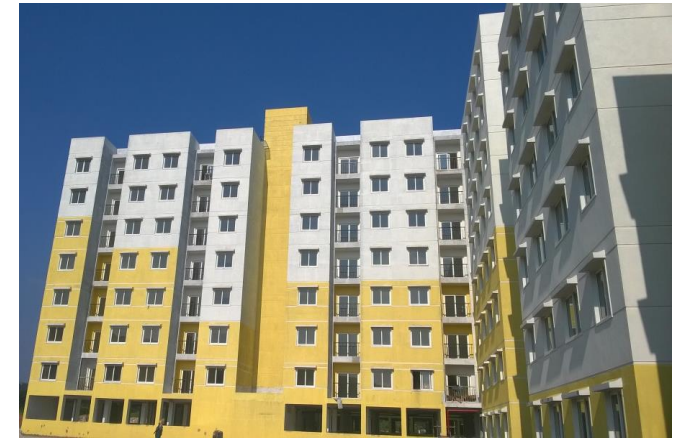
Nova Phase I Block C1 (Mar'16)
