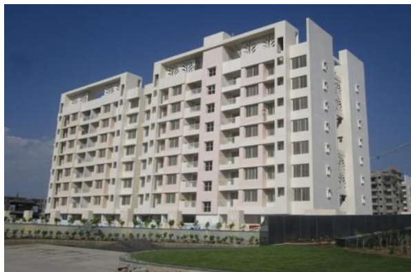
Bloomdale Phase IA, IB & IC Handovers in progress
