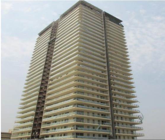
Luminare - Tower A (Mar' 18)
