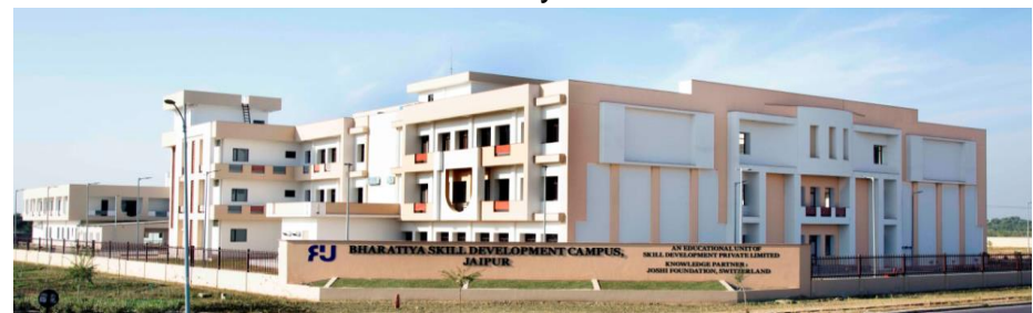
Bharat Skill Development University facility in DTA
