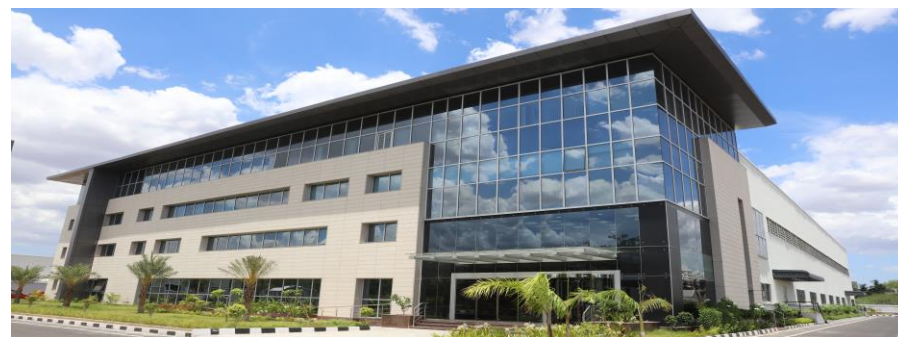
Dorma Kaba facility in DTA
