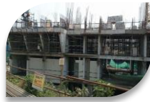
Alcove (Under Construction)
