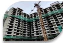
Happinest Kalyan (Under Construction)
