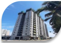
Lakewoods, Chennai (Under Construction)
