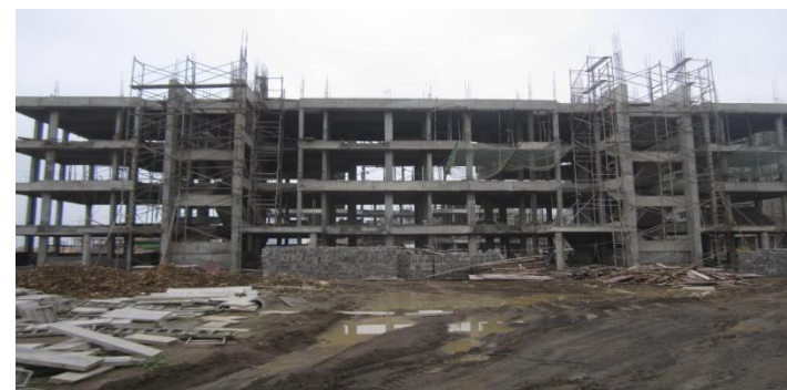
Phase IC – Duplex House 7,8( Sep'13)
