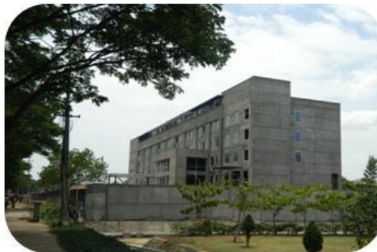
HolidayInn Express (Under construction)
