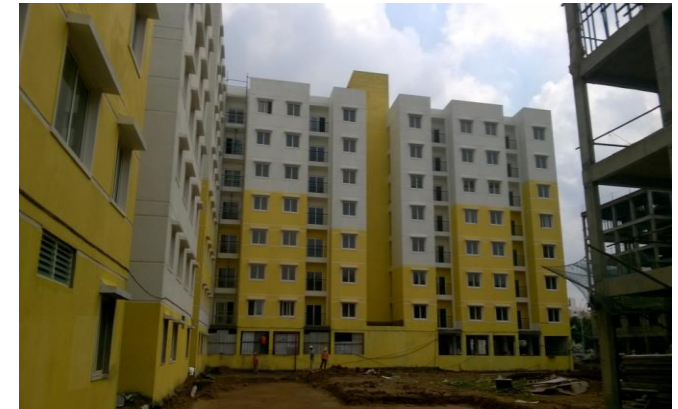
Nova Phase I Block C2 (Sep'15)
