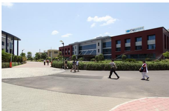
Capgemini facility, IT SEZ
