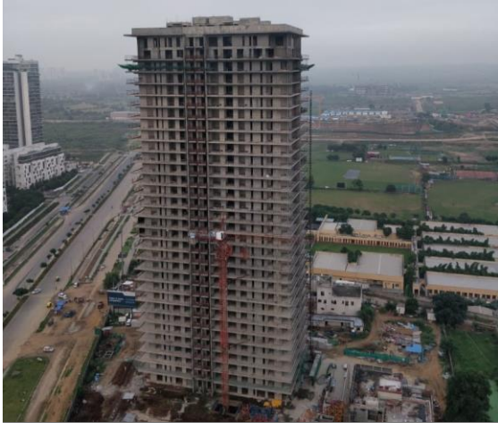
Luminare - Tower C (Sept'18)
