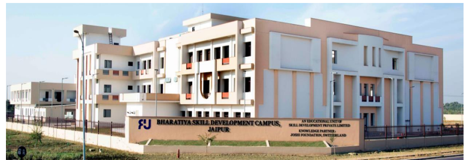
Bharat Skill Development University facility in DTA
