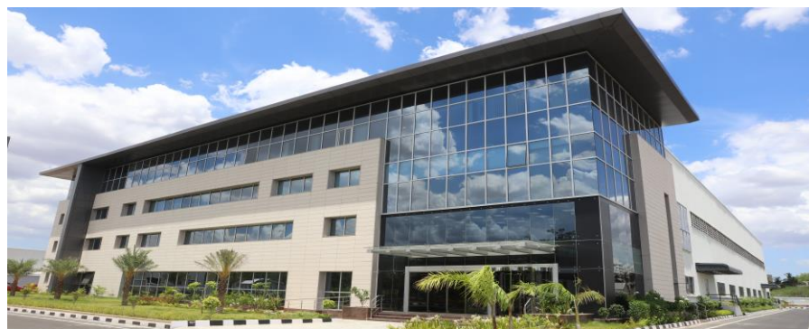
Dorma Kaba facility in DTA
