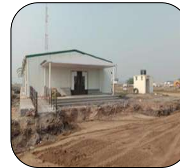
Under Construction Site
