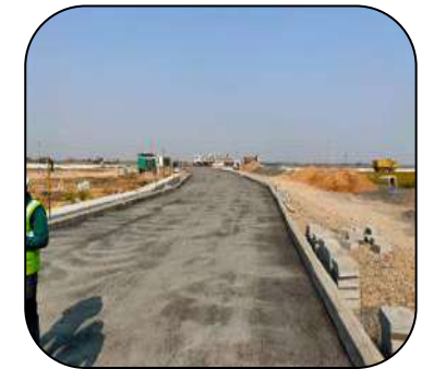
Under Construction Site
