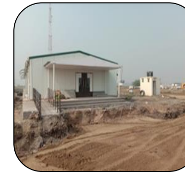
Under Construction Site
