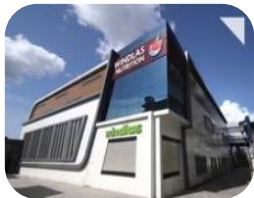
Dehradun Plant 1 commenced operations in 2001
