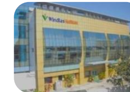
Dehradun Plant 4 commenced operations in 2009
