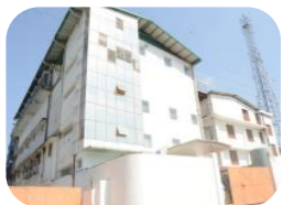
Dehradun Plant 2 commenced operations in 2014
