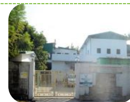
Dehradun Plant 3 commenced operations in 2018
