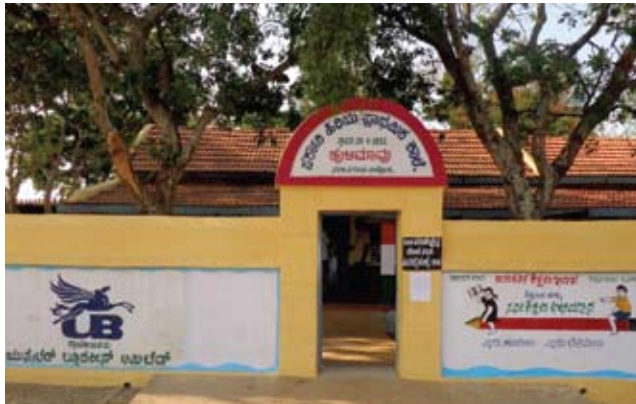
Primary school refurbished in Nanjangud, Karnataka.
