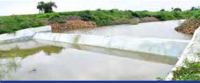
Check Dam construction in Kondapur Block, Telangana
