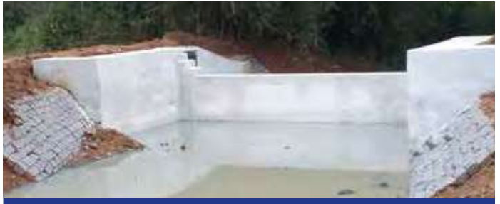
Check Dam Construction in Nelamangala, Karnataka
