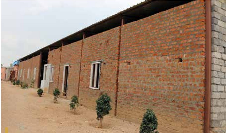
Contributed in building Orphanage home at Nalgonda which is under construction
