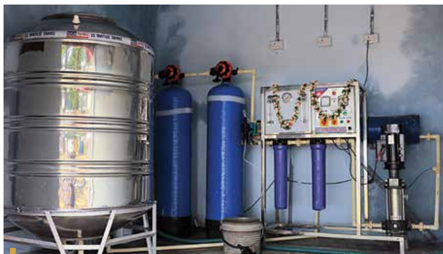
Built a water purification plant at Toopranpet
