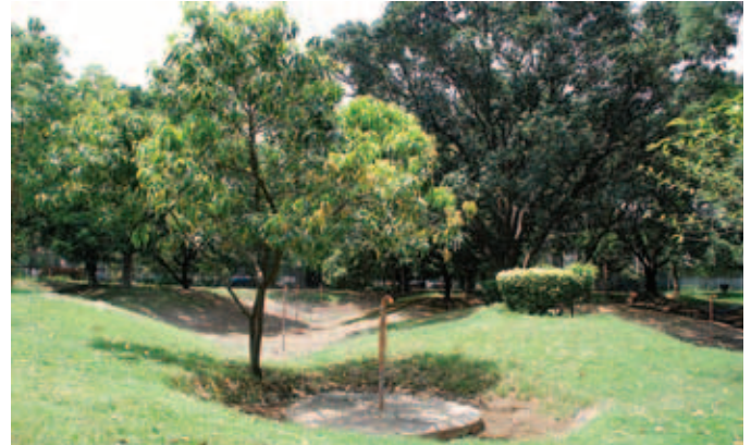
LAGOONS TO CAPTURE RAINWATER AT GURGAON FACILITY
