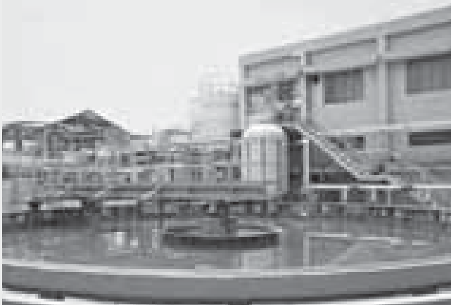
Effluent treatment plant at Gurgaon
