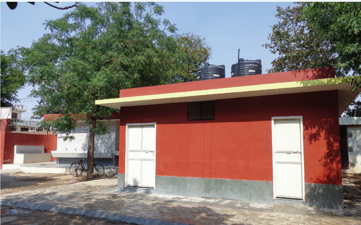
Construction of separate toilet blocks for boys and girls in Government schools
