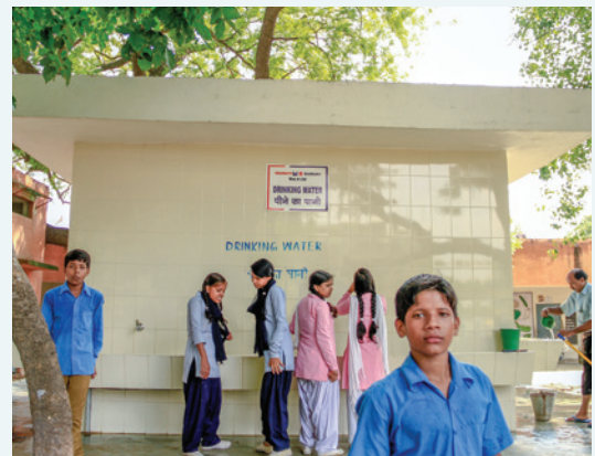
New drinking water facility constructed with bigger tank capacity
