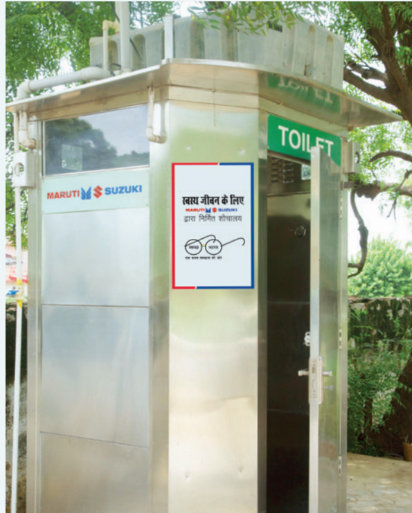
Installed stainless steel community toilets in villages
