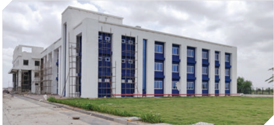
School in Sitapur, Gujarat under construction
