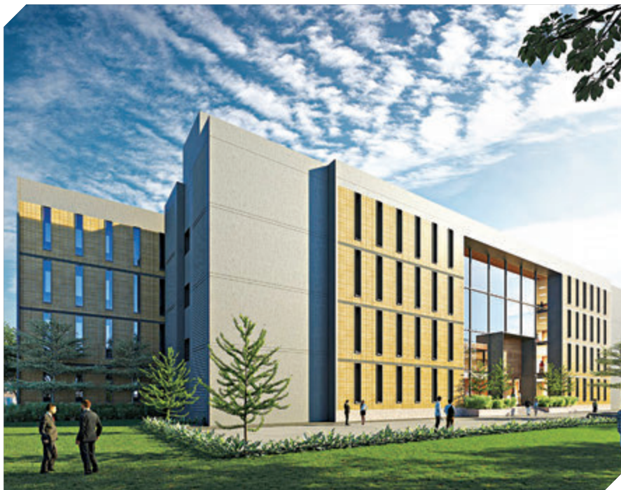
Representative photo of multi-specialty hospital under construction in Sitapur, Gujarat
