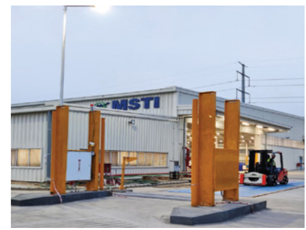
A view of MSTI facility
