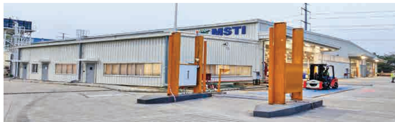
A view of MSTI facility
