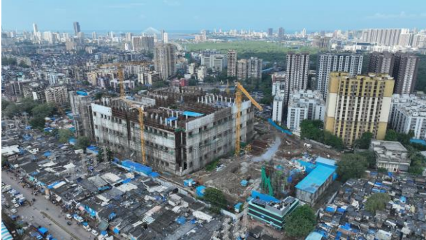
Dharavi WWTP India's First multi -storied WWTP
