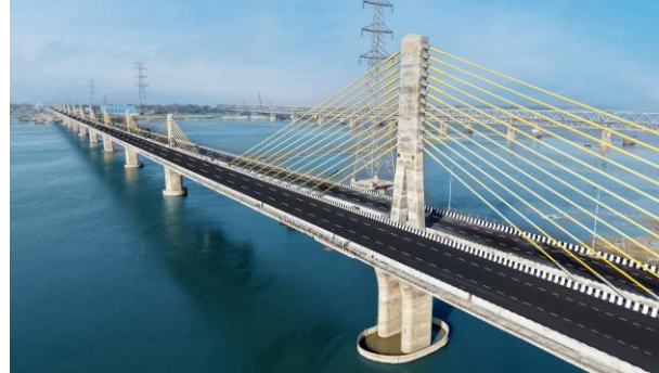
Auntha-Simaria Bridge India's widest extra-dosed cable-stayed
