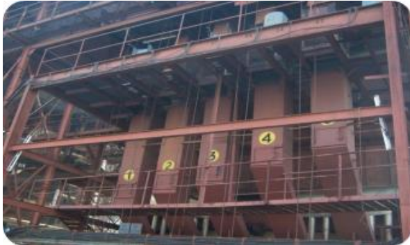
Bagasse Silos & Feeders of Boiler
