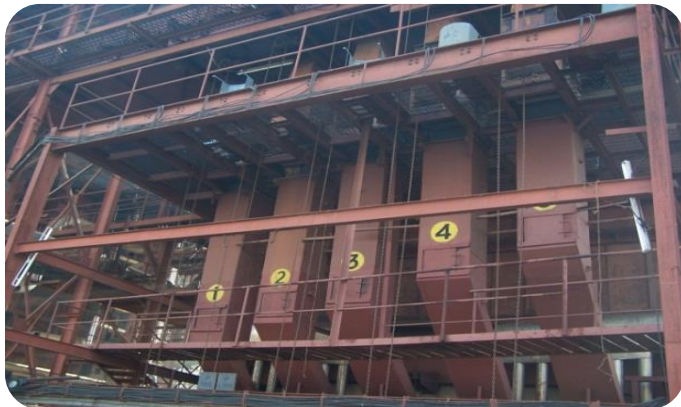
Bagasse Silos & Feeders of Boiler
