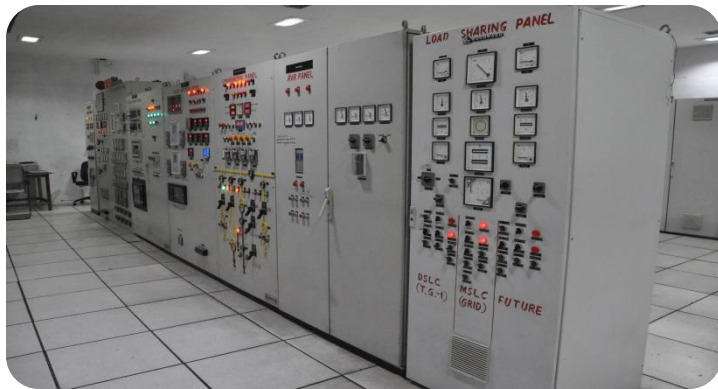
Cogeneration Control Panel
