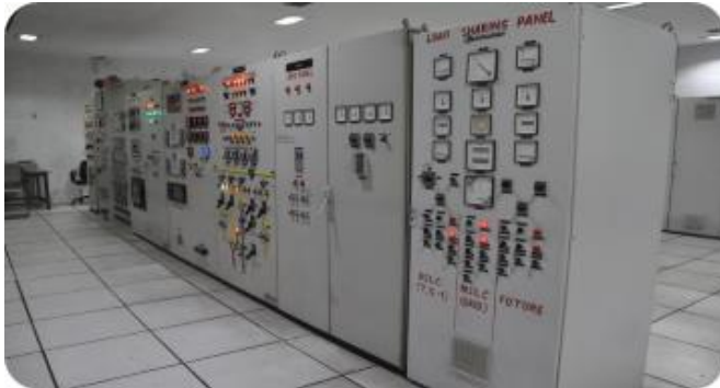
Cogeneration Control Panel
