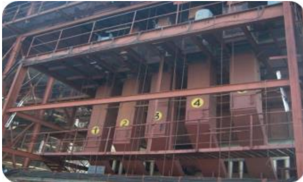
Bagasse Silos & Feeders of Boiler
