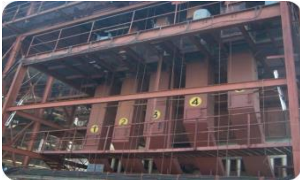
Bagasse Silos & Feeders of Boiler
