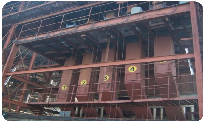
Bagasse Silos & Feeders of Boiler
